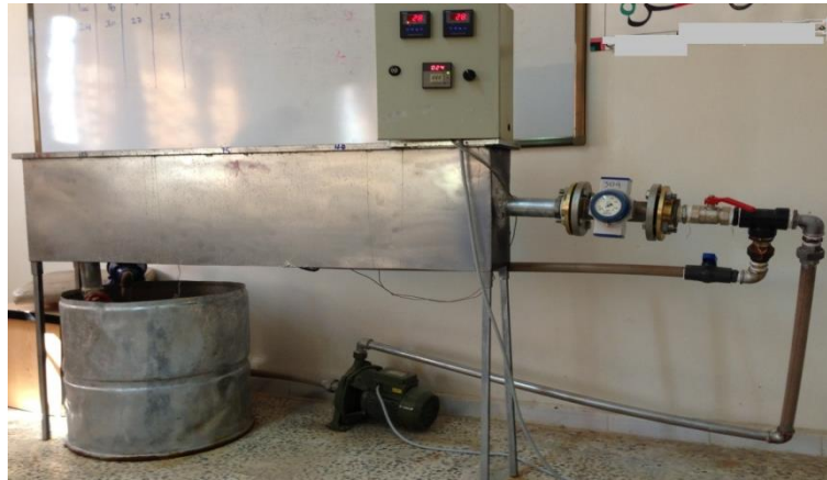
Figure 1.6 water system to examine the performance of heat transfer setup.
